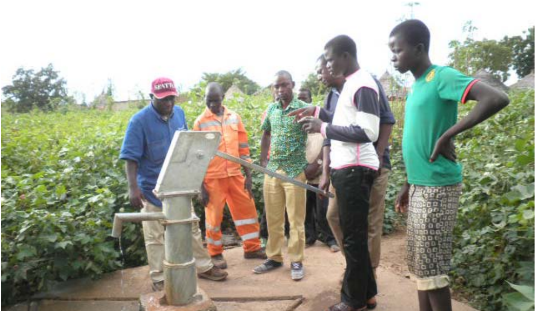
Borehole built by CIMENCAM near Bidzar (photo Norbert BOUBA)
