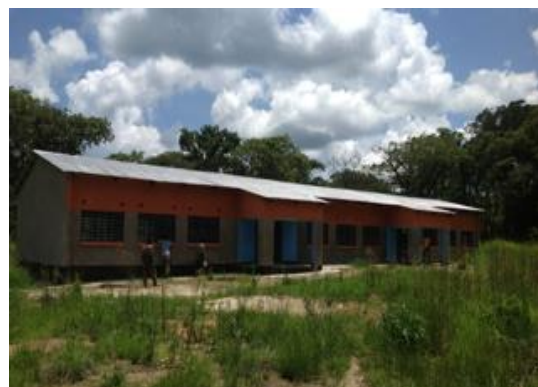
Figure 8: Completed School as 21st January 2013, but not commissioned
